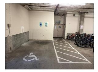
An accessible parking space must be located on a surface that does not exceed a two percent grade (equivalent to a slope of 1:48) in all directions. Additionally, covered parking facilities such as parking garages must have a minimum vertical clearance of 98 inches over each van accessible space.
